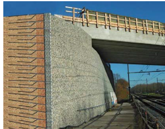
Figure 8: Bridge abutment with gabion facing [7]
