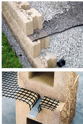
Figure 4: Mechanical connection (pin through) and Frictional connection (lip of block) of geogrid fabric with modular blocks [5]
