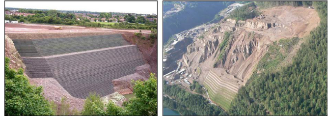
Figure 7: Geogrid fabric reinforced steep slopes [7]
